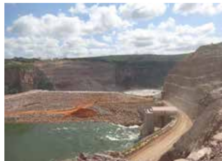
Resin injection for clogging water intake in the diaphragm walls.
