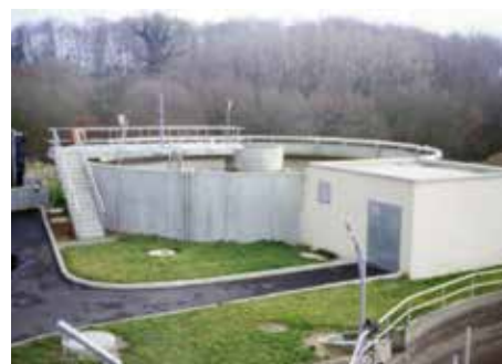
Wastewater Treatment Plant Hassasna.
