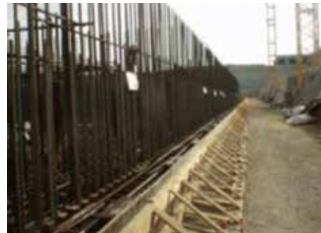
Treatment of joint protection.
