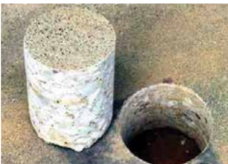
Execution of drilling in reinforced concrete slabs.
