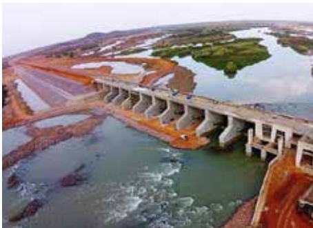
Treatment of concrete and waterproofing.
