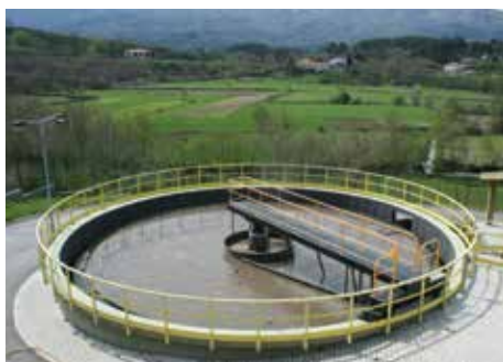
Effluent waters treatment plant.
