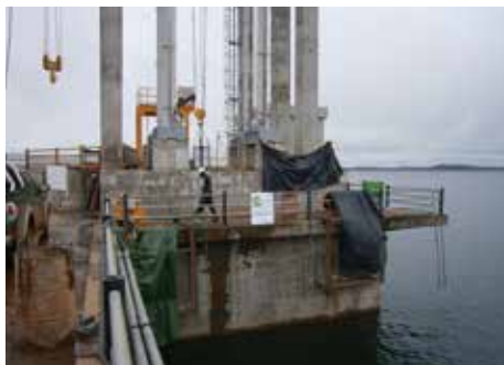
Injection resins tower water outlet.
