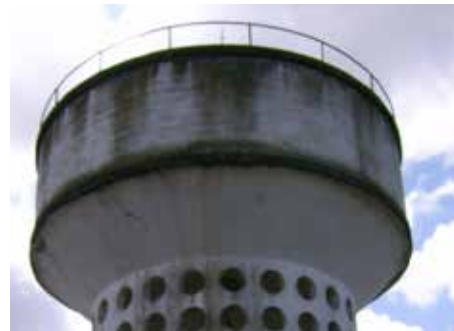
Treatment of concrete and waterproofing of potable water reservoir.
